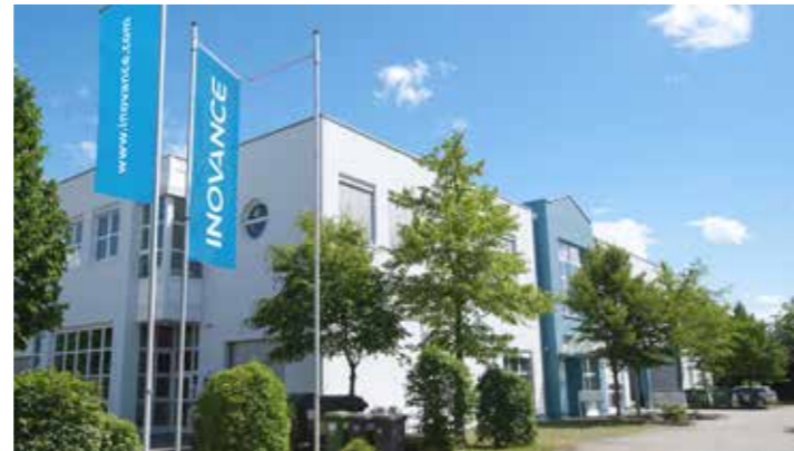
Inovance Technology Europe's headquarters in Stuttgart, Germany
